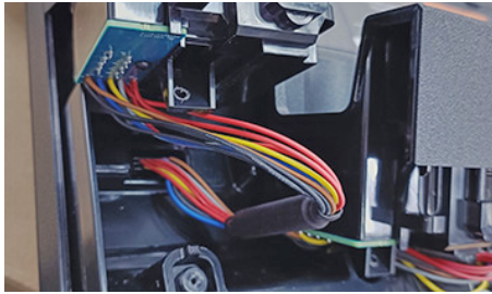
Figure 28: Cable Removal for Each Pocket Insert
